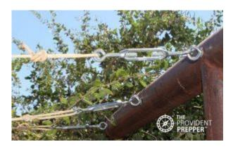
The supports for our clothesline are built from two pipes welded together, creating a T shape. The supports are spaced about 15 feet apart.
